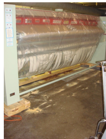
New Finish Master 2400 Installation
